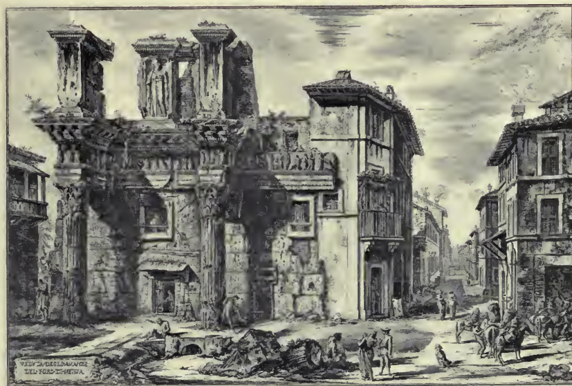
THE FORUM OF NERVA. INTERIOR OF ENCLOSURE WALLS WITH THE TWO HALF-BURIED CORINTHIAN COLUMNS. 95, II
